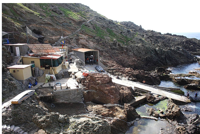
The complex of buildings on Selvagem Grande built for the Naval Police and their large RIB Dr Frank Zino
